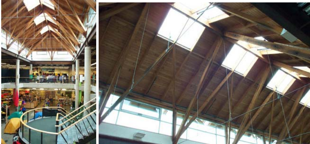
Figure 8: Mountain Equipment Coop, Toronto, Stone Kohn and Vogt Architects Indoor Environmental Quality: Credit 8 Daylighting – use of glazing to daylight the space can increase heat loss (winter) or heat gain (summer) if not properly detailed and specified
