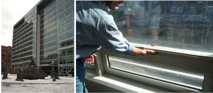
Figure 11: Innovation and Design Process: Caisse de Depots et Placements, Montreal Double skin wall construction.
