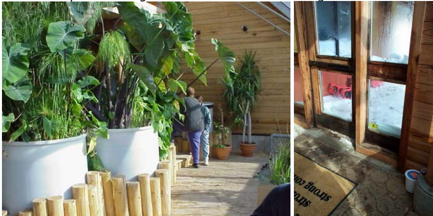
Figure 3: YMCA Environmental Learning Centre, Charles Simon Architect Water Efficiency: Credit 2 Innovative Wastewater Technologies: Living Machine™ – adjacent doors suffering from deterioration due to the high moisture content of the room
