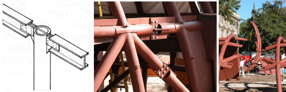
Figure (left): Detail from Ching of a type of tube to WF connection
