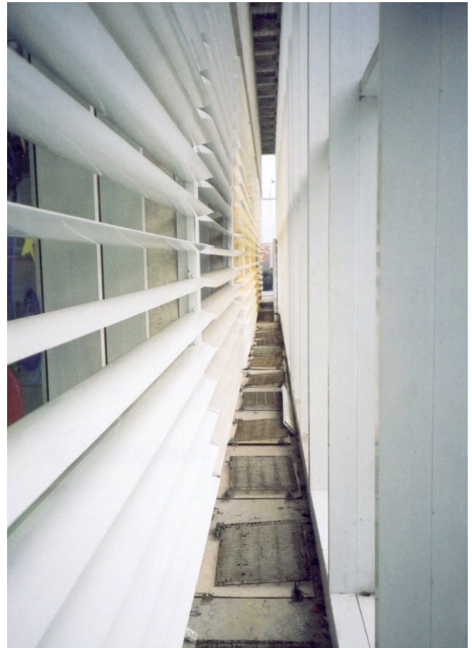
Photos of the interior of the wall cavity and clouding of the exterior skin. Detail photo of skin clouding taken by Terri Meyer-Boake.
