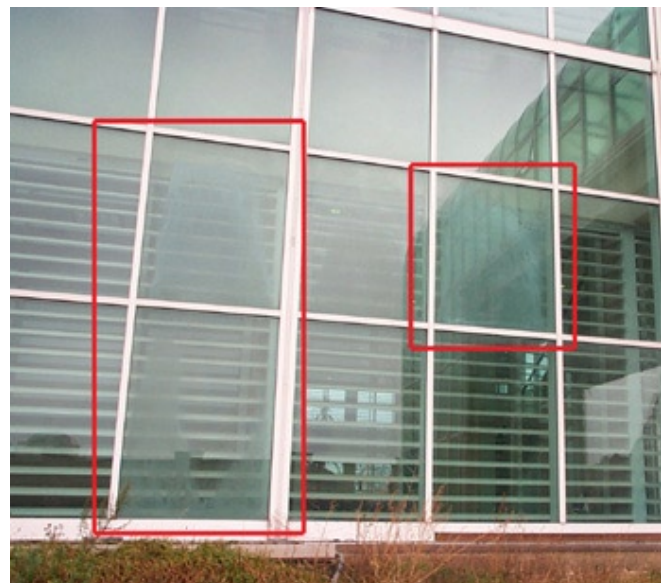
Photos of the interior of the wall cavity and clouding of the exterior skin. Detail photo of skin clouding taken by Terri Meyer-Boake.
