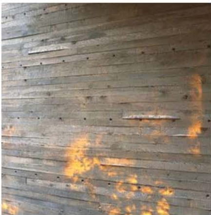
20. Wood-formed concrete embeds the project into the surrounding site. The use of the wood forms makes the concrete appear heavy and light.
