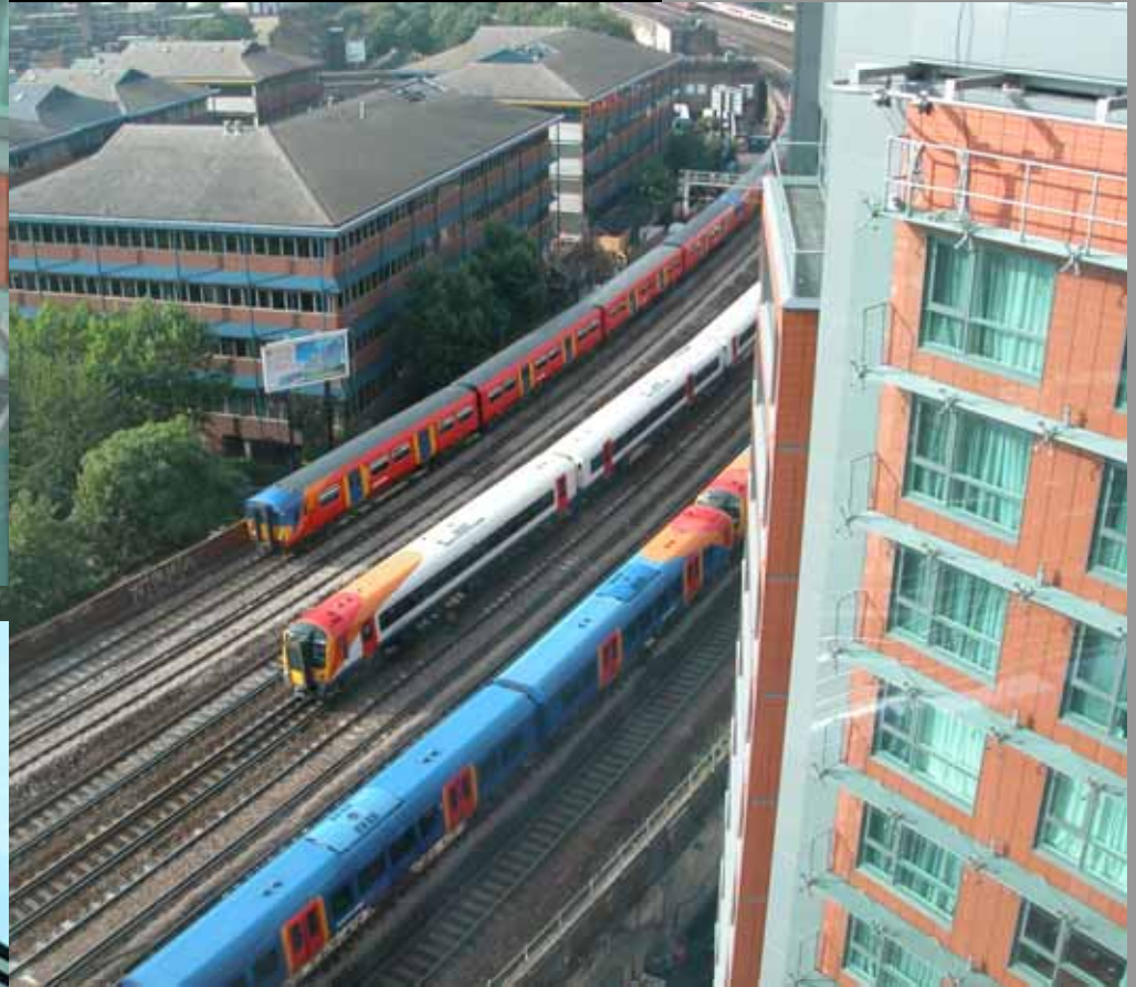
London: An extra layer of glazing creates an acoustic buffer against rail noise, while still allowing operable glazing units behind.
