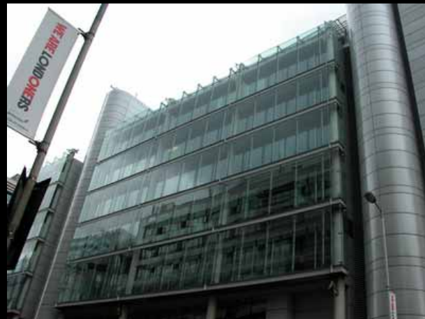
Helicon, Finsbury Pavement
