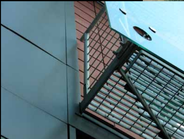
London: An extra layer of glazing creates an acoustic buffer against rail noise, while still allowing operable glazing units behind.
