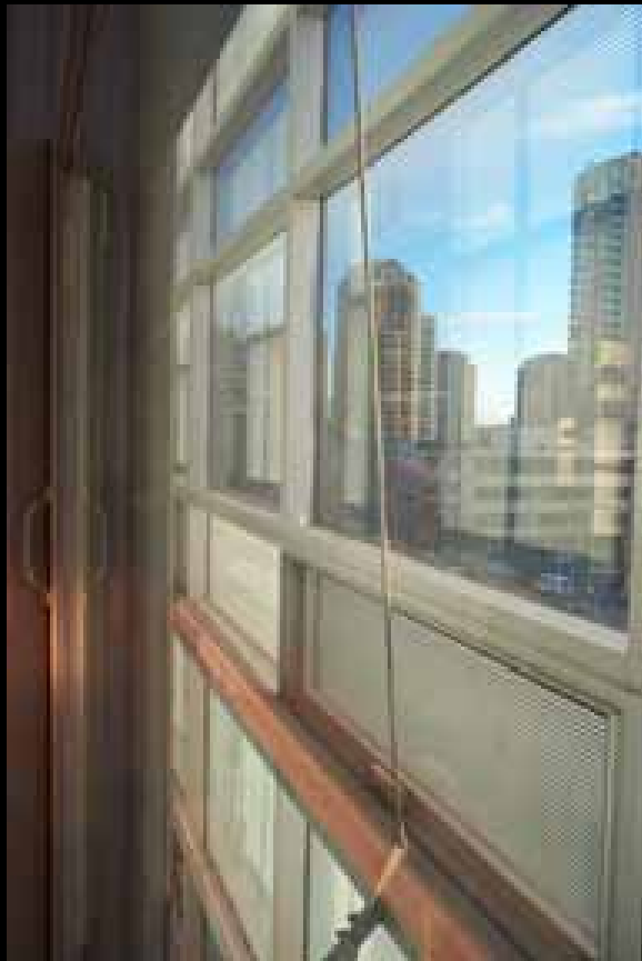
Views inside cavity
