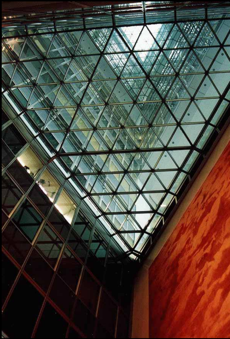
Views through central atrium
