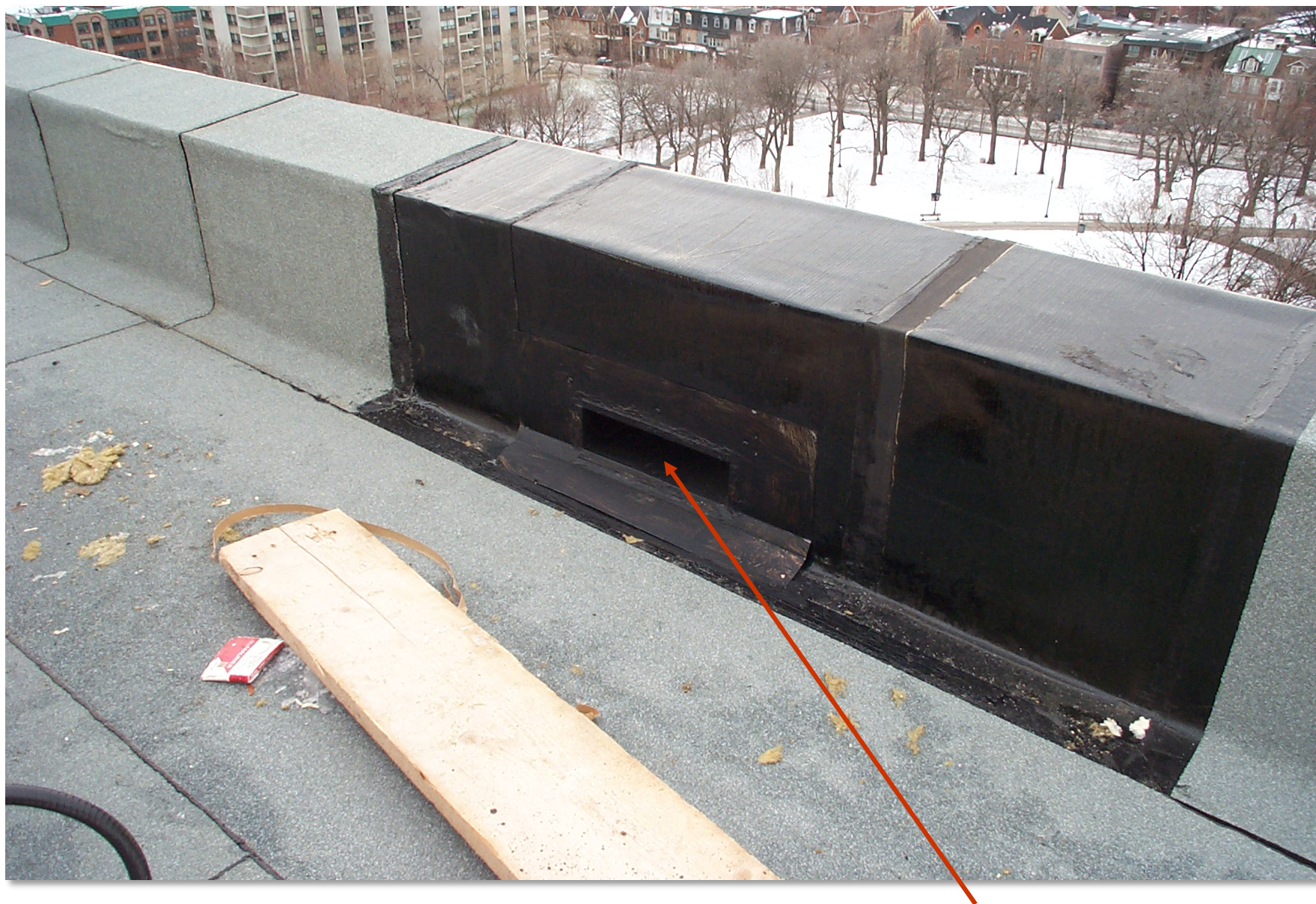
Detail at parapet. Note water overflow opening.
