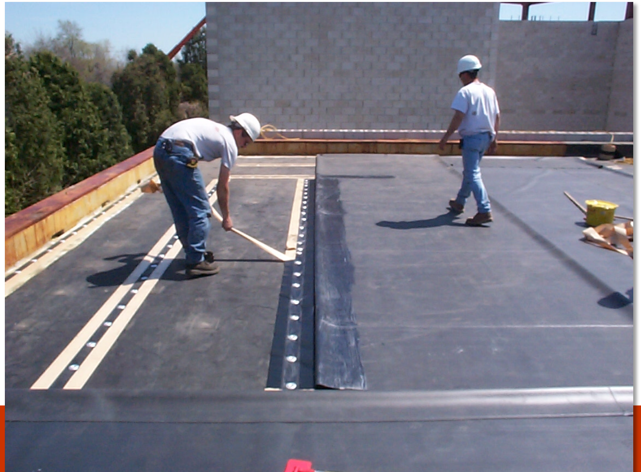
Mechanical fastening strips and an EPDM roof
