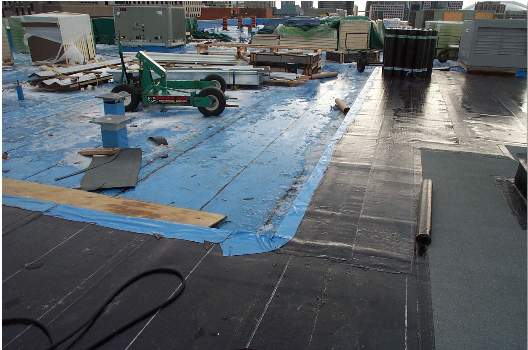
This is a multi-ply installation. The black being the base layer and the grey the more durable top layer. The insulation is beneath the black layer.
