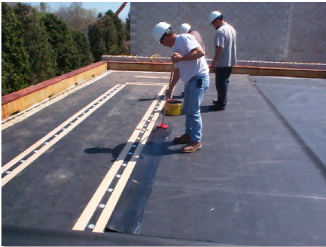
Mechanical fastening strips and an EPDM roof
