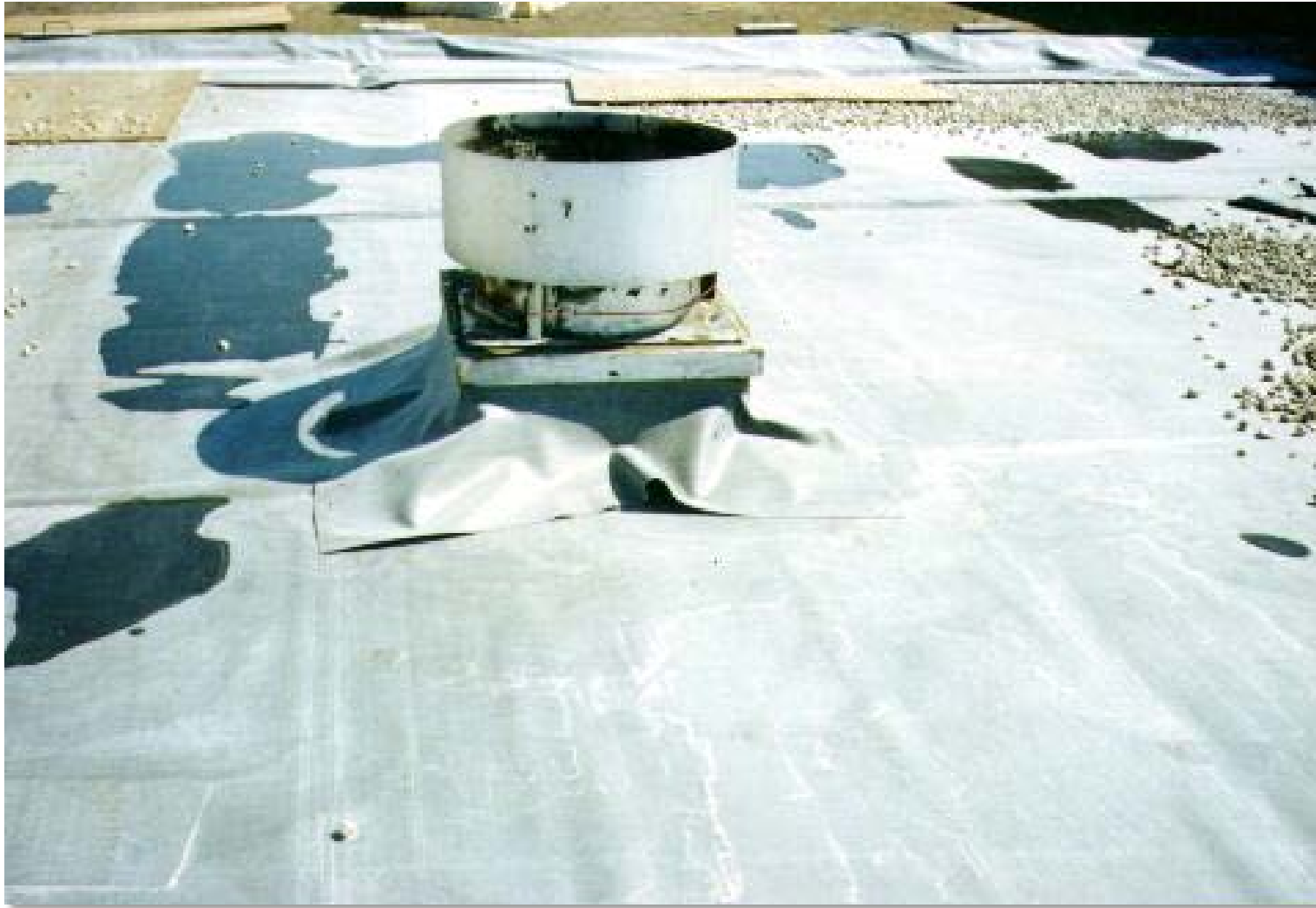
EPDM - loose laid and ballasted
