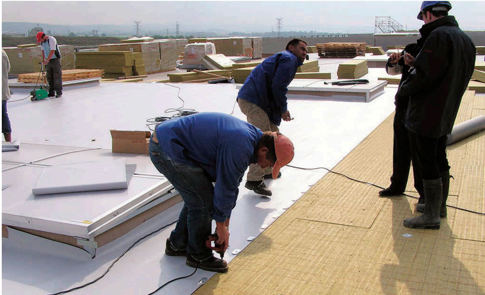
Roofing membrane is being installed over the dense/rigid rockwool insulation to protect it from moisture.
