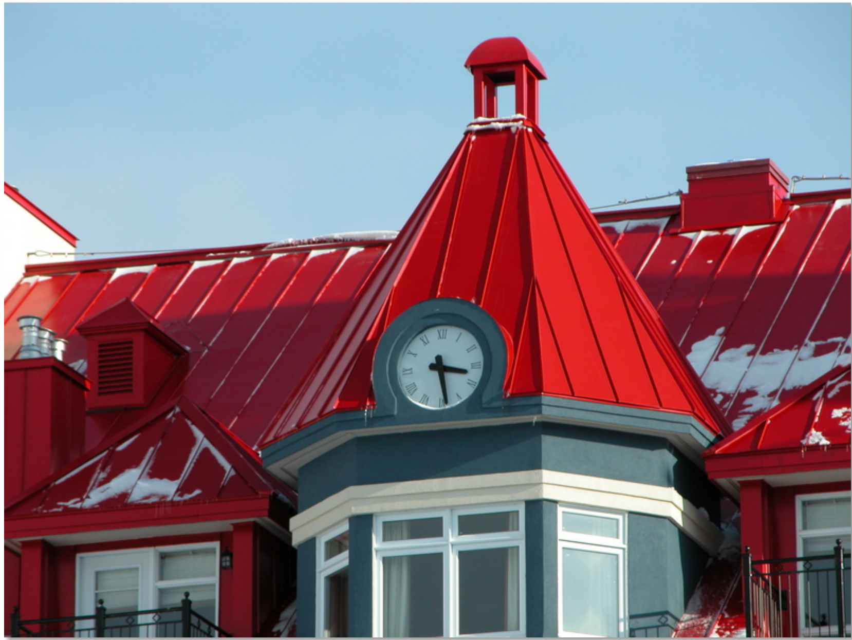
Contemporary Standing seam metal roof
