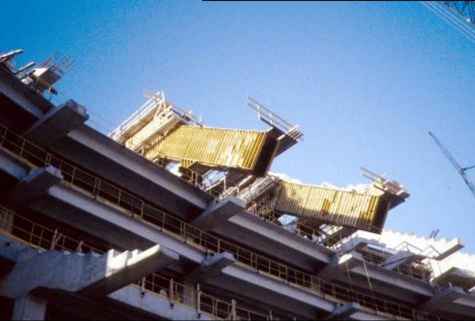
Insulated concrete forms for cold weather pouring at Skydome (Rogers Centre) Toronto
