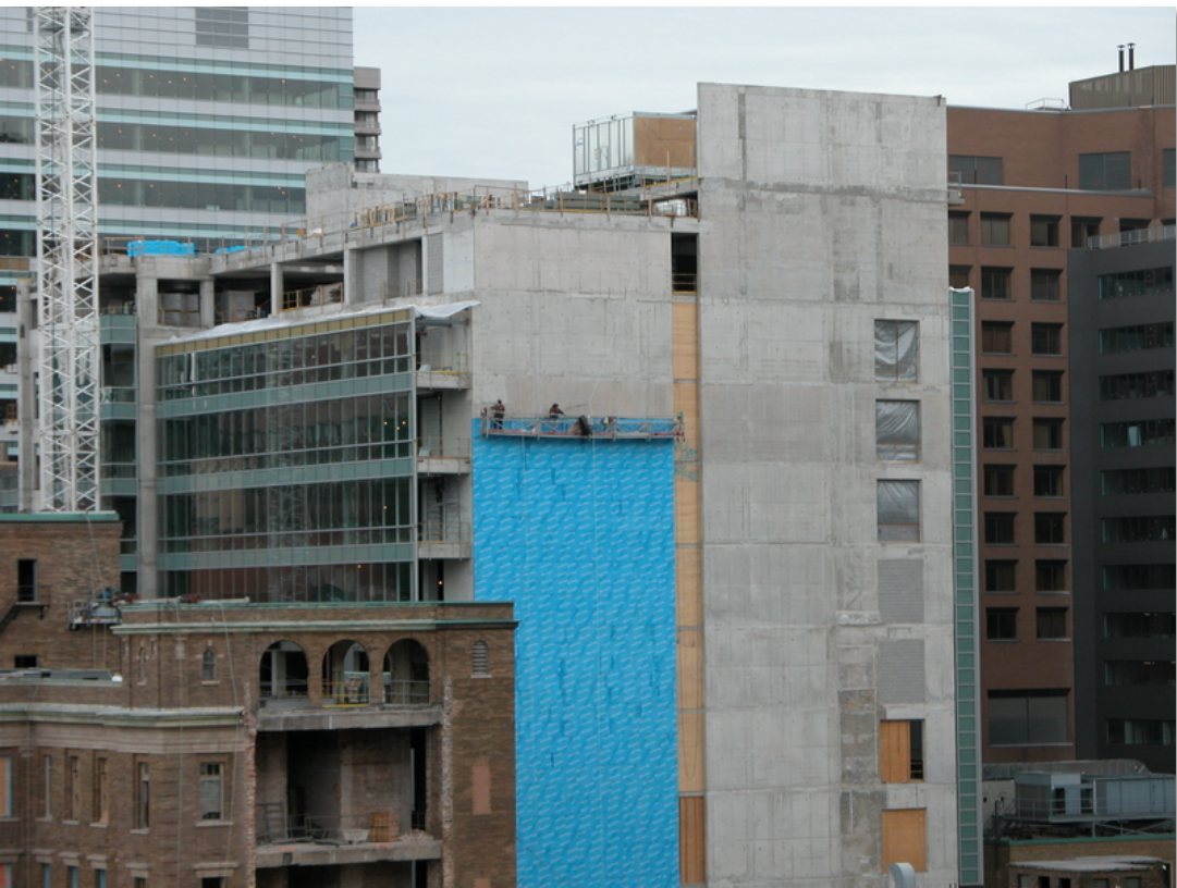
Installation of Blueskin on Mars in downtown Toronto.
