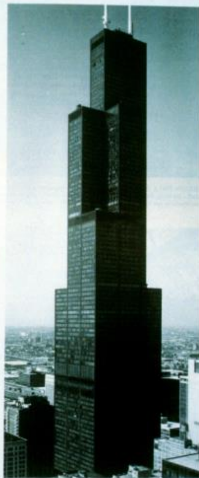
Crystal Palace would have been too heavy for its cast-iron columns; now steel beams make such buildings possible. At right is Skidmore, Owings & Merrill's Sears Tower, built out of stacked modular units.
