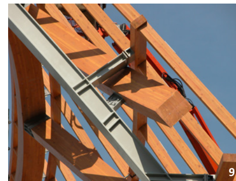
9 Composite structural systems require higher levels of coordination. The tolerances and construction practices of the other material must be taken into account.
