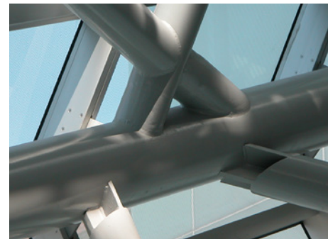
125 Complex connections using square HSS members are very difficult when it comes to alignment. Circular members are more forgiving. This connection is located on a high-level skylight, so the alignment issue is not really visible.
