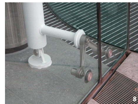
8 Specialty glazing systems require tighter tolerances and a higher level of Fit on a project.
