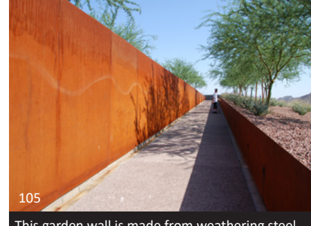
105 This garden wall is made from weathering steel. Although durable in appearance, you can see the destructive markings on the surface made by users of the space. It is essential to detail these types of installations so that the run-off water does not stain surfaces below the wall.
