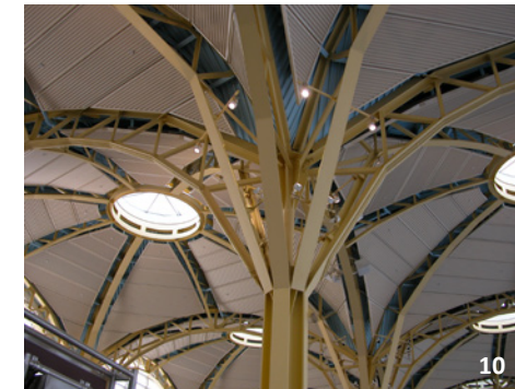
10 Two different steel trees: one created using W shapes to create a very textured appearance; the other using mechanical pipe and specialty castings and striving for a seamless appearance using a high gloss finish. AESS specifications must be tailored to the overall design intentions of each individual project as they are all somewhat unique.
