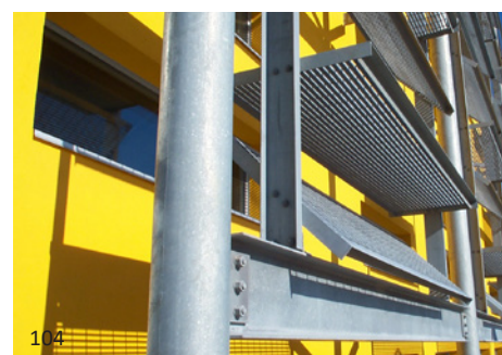
104 Galvanizing is very popular as a finish, but remember that its basic purpose is as a corrosion-prevention coating. The nature of the finish will not be consistent from batch to batch.
