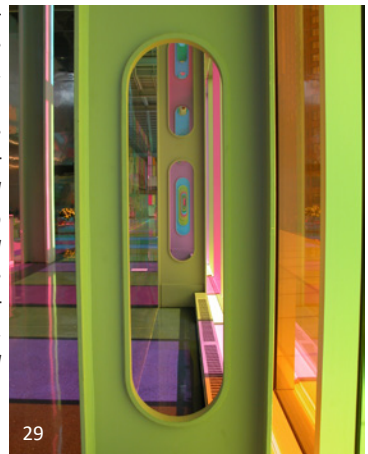
The Palais des Congrès in Montreal uses specialty W sections with trimmed cutouts. Although the steel is all painted grey, and intumescent coatings are used, the coloured light through the curtain wall gives additional texture to this expression of steel.
