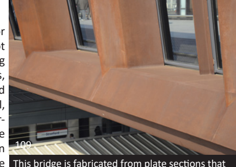
109 This bridge is fabricated from plate sections that have been custom bent then welded together to create larger sections. The welds are left as is - high quality welding acceptable as part of the more rugged appearance of this product.
