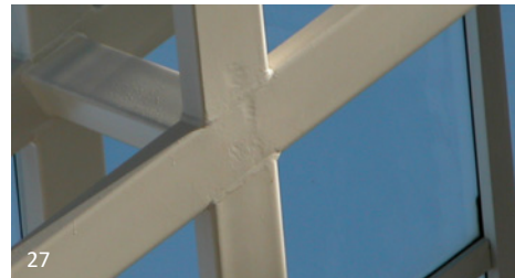
Edmonton City Hall: The trusses that support the pyramidal glass roof are created using square HSS sections. The viewing distance varies but is typically greater than 6 metres, even from the upper levels. An up-close inspection reveals many inconsistencies that are reasonable to leave “as is” due to the view distance. The extra expense to fill, grind and carefully align the members would be lost on users of the building.
