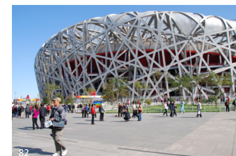
Complex geometry, odd angles and extremely heavy elements add a cost premium to this project. The level of form, fit and finish on this project is exceptionally high. In the UK a high level of tradition of AESS has been established which has resulted in a highly skilled labour force.
