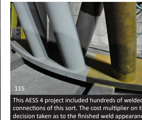
115 The large “wishbone” sections used at Pearson International Airport were special enough to warrant a full scale mock-up. The size and cost of the mock-up were such that it was made to be incorporated into the project. Although there may be slight differences in the final design, these are imperceptible in situ. Top image: Walters Inc.
