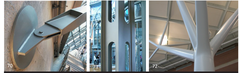
Fig. 4.3B Surfaces filled and sanded. These three examples show very different applications of AESS 4 whose details require extra care and high-level consistency such that any and all imperfections are filled (typically with body filler) and sanded prior to the application of the finish coating. It is particularly important in the left and right images where a glossy finish is to be applied.
