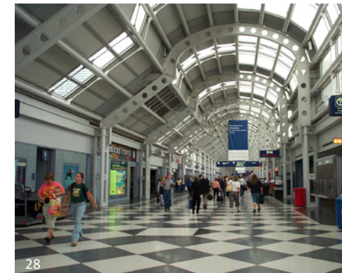
O'Hare International Airport in Chicago was the first airport to use AESS. Much of the steel is well within range of view and touch. A variety of steel shapes and connection types have been used. The complex nature of the sections and connections called for a tighter sizing tolerance and even finish application.
