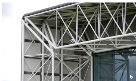
6 The Sainsbury Centre for the Performing Arts was designed and constructed by Norman Foster in 1977. The British High Tech movement brought exposed structural steel to the forefront of design, and with it an array of issues that had not been part of architectural discourse for more than a century. The project used round HSS members and a structure that was expressed on both the exterior and interior of the building.
