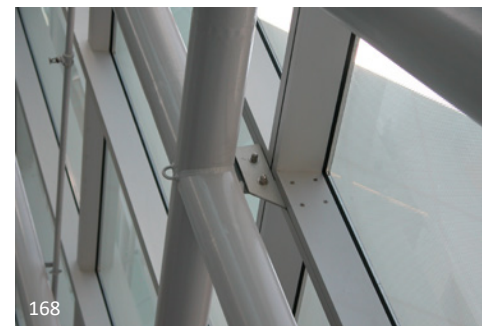
168 This tubular steel framing system connects to the sloped curtain wall in a more traditional fashion with slim line supports being fairly concealed behind the profile of the HSS sections.
