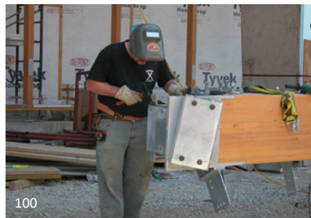
100 The base connectors for these hybrid steel and glulam timber members have been fabricated from galvanized steel. The position of the connector in the building put it at greater risk of moisture exposure, so painted steel was not desired.
