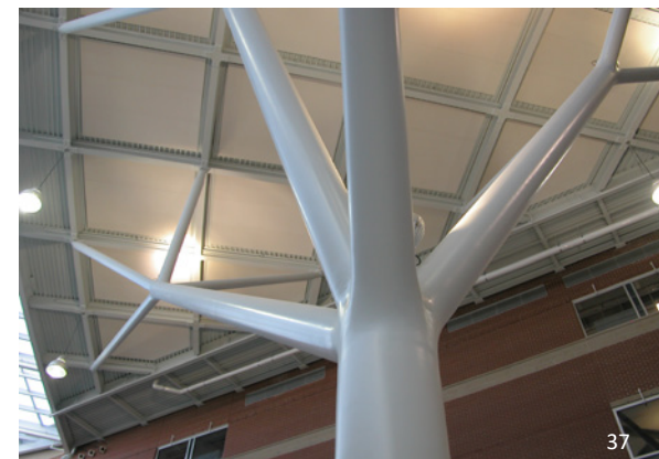
University of Guelph Science Building Courtyard uses special castings to cleanly join mechanical pipe and a structural tree that stands in the centre of the courtyard. The requirement for a seamless transition from the pipe to the casting required unusual welding and filling of the connection, as well as grinding of the surface of the casting so that its normal textured finish would match the surface condition of the adjacent pipe.
