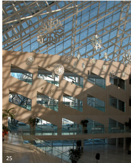
Edmonton City Hall: The trusses that support the pyramidal glass roof are created using square HSS sections. The viewing distance varies but is typically greater than 6 metres, even from the upper levels. An up-close inspection reveals many inconsistencies that are reasonable to leave “as is” due to the view distance. The extra expense to fill, grind and carefully align the members would be lost on users of the building.
