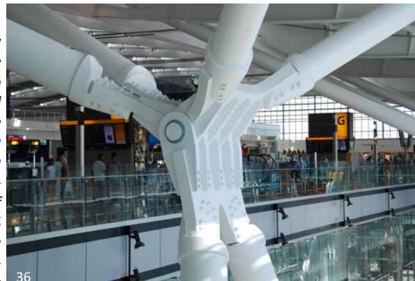
Heathrow Terminal 5 in London, England by Sir Richard Rogers Architect uses a range of AESS Category types throughout the terminal. These specialty connections use a combination of custom work for the central hinge, castings to connect the ends of the large HSS supports and truss members to the hinge, and showcase level of fabrication and finish for the legs/column supports. You need to be flying British Airways to come across this steel!
