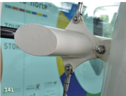
141 The cross sectional shape of this elliptical tube was chosen as part of a slender glazing support system in an airport.
