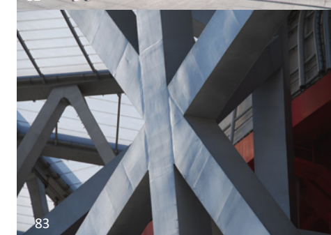
The scale and complexity of this welded project meant high cost premiums and additional fabrication and erection time. The project was additionally complicated as a result of fabrication and erection in China. There is far less AESS work that is routinely made a part of Chinese construction, so skilled labour can be an issue. The sections were created using plates and, given varied lighting conditions, many of the welds were visible. The overall aesthetic of the project could accommodate this level of texture.
