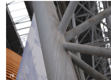
The quality of the ironwork, welding and finish on this museum in inner China was extremely low. The welds were sloppy. The intumescent coating appeared to have been applied when the project was still open to the weather, resulting in dirt streaks down all of the members. In spite of the overall creative energy of the design of the building, the lack of care in workmanship due in part to problems in communication, supervision and understanding of the role of AESS undermined this installation.
