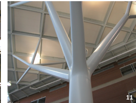
10 Two different steel trees: one created using W shapes to create a very textured appearance; the other using mechanical pipe and specialty castings and striving for a seamless appearance using a high gloss finish. AESS specifications must be tailored to the overall design intentions of each individual project as they are all somewhat unique.
