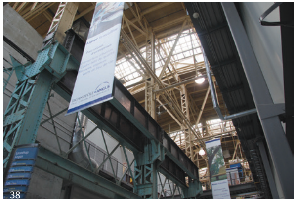
Angus Technopole, Montreal is a unique reuse application of a former locomotive shop as offices and commercial space. The riveted steel was left “as is”, with minimal cleaning and no repainting, to preserve the original look and feel of the building. Where new steel is required in this project, a custom specification is required in order to make it fit into the aesthetics of the old building.
