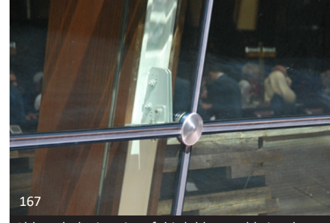
167 Although the interior of this lobby would give the appearance of being supported in heavy timber, here we can see that the framing is steel with wood cladding. This permits the connection of spider connectors to the steel structure hidden inside.
