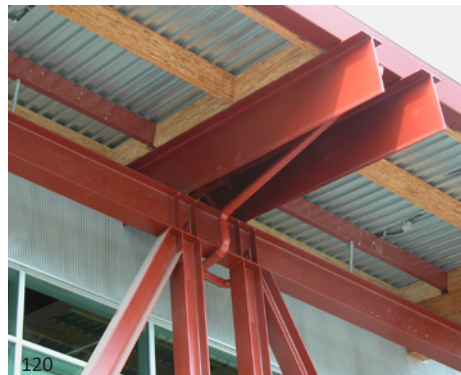
119 This project included a high level of texture using standard structural shapes, and so bolting was chosen to connect the welded elements.
