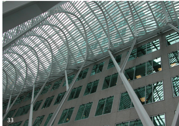
Brookfield Place in Toronto by Spanish Architect Santiago Calatrava uses AESS 4 quality fabrication and finish on the lower portion of the tree supports in the Galleria space. All of the members use welded connections with a hand-smooth finish and no apparent blemishes. Given the articulation and complicated geometry, tolerances for this structure were even less than one-half standard fabrication. The “canoes” that form the support for the skylight are well above view level and use a combination of welding and bolting.
