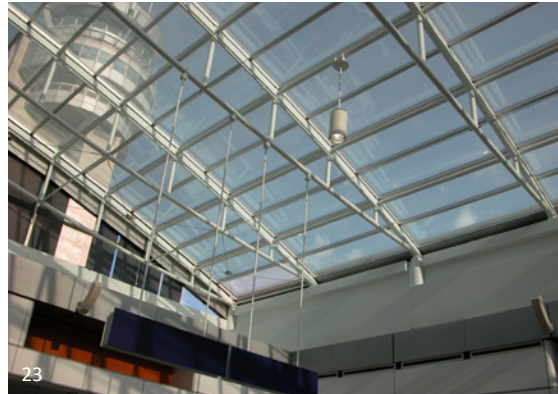
Pierre Elliott Trudeau Airport, Montreal: The trusses supporting this skylight are quite characteristic of AESS 2 type steel. The viewing distance is over 6 metres but the design needs something more than a standard joist or truss. The detailing is simple, and the viewer is not close enough to see the texture of the connection, only the form of the truss.
