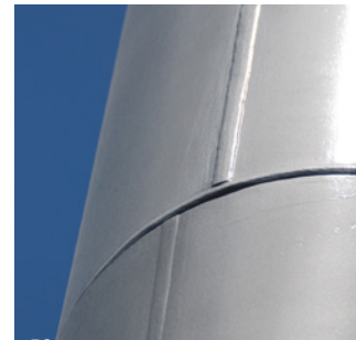
59 Fig. 3.3A The natural weld seams on these connecting HSS sections may have been better detailed if they had been aligned.
