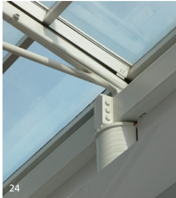
Pierre Elliott Trudeau Airport, Montreal: The trusses supporting this skylight are quite characteristic of AESS 2 type steel. The viewing distance is over 6 metres but the design needs something more than a standard joist or truss. The detailing is simple, and the viewer is not close enough to see the texture of the connection, only the form of the truss.
