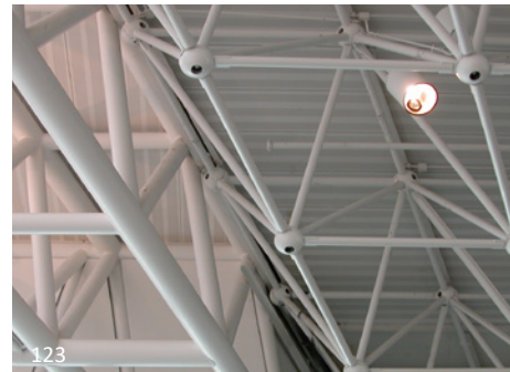
122 Although the overall form of this box truss appears complex, the 100% welded connections have been designed with simple geometries.
