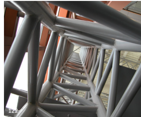
119 This project included a high level of texture using standard structural shapes, and so bolting was chosen to connect the welded elements.
