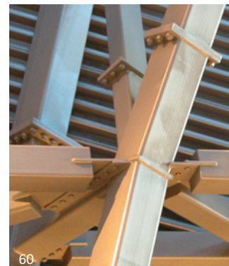
60 Fig. 3.3B The seams on the square HSS sections have been aligned and, even on the outside face of the connection, seem in keeping with the overall design intention.
