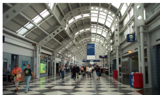
7 In its article on Architecturally Exposed Structural Steel Construction in Modern Steel Construction (May 2003), AISC cited the roots of the current trend of exposed steel and transparency in design to the Chicago O’Hare United Airlines Terminal designed by Helmut Jahn between 1985 and 1988. Indeed, airport architecture has succeeded in pushing the use of exposed steel to incredible heights.
