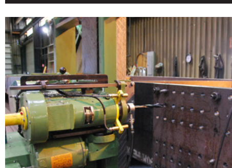
150 The drilling of holes is an automated process. This ensures that holes are drilled with very even spacing on each member.
