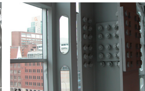
62 Fig. 3.4 This column splice is within touching range, but the column flanges do not line up and the connection plate seems too short.
