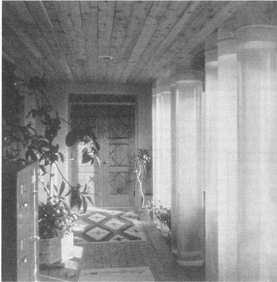
**Figure 7.9d** A Trombe wall can consist of vertical tubes filled with water. The tubes can be opaque, translucent, or transparent. (Courtesy of and © Solar Components Corporation.)
