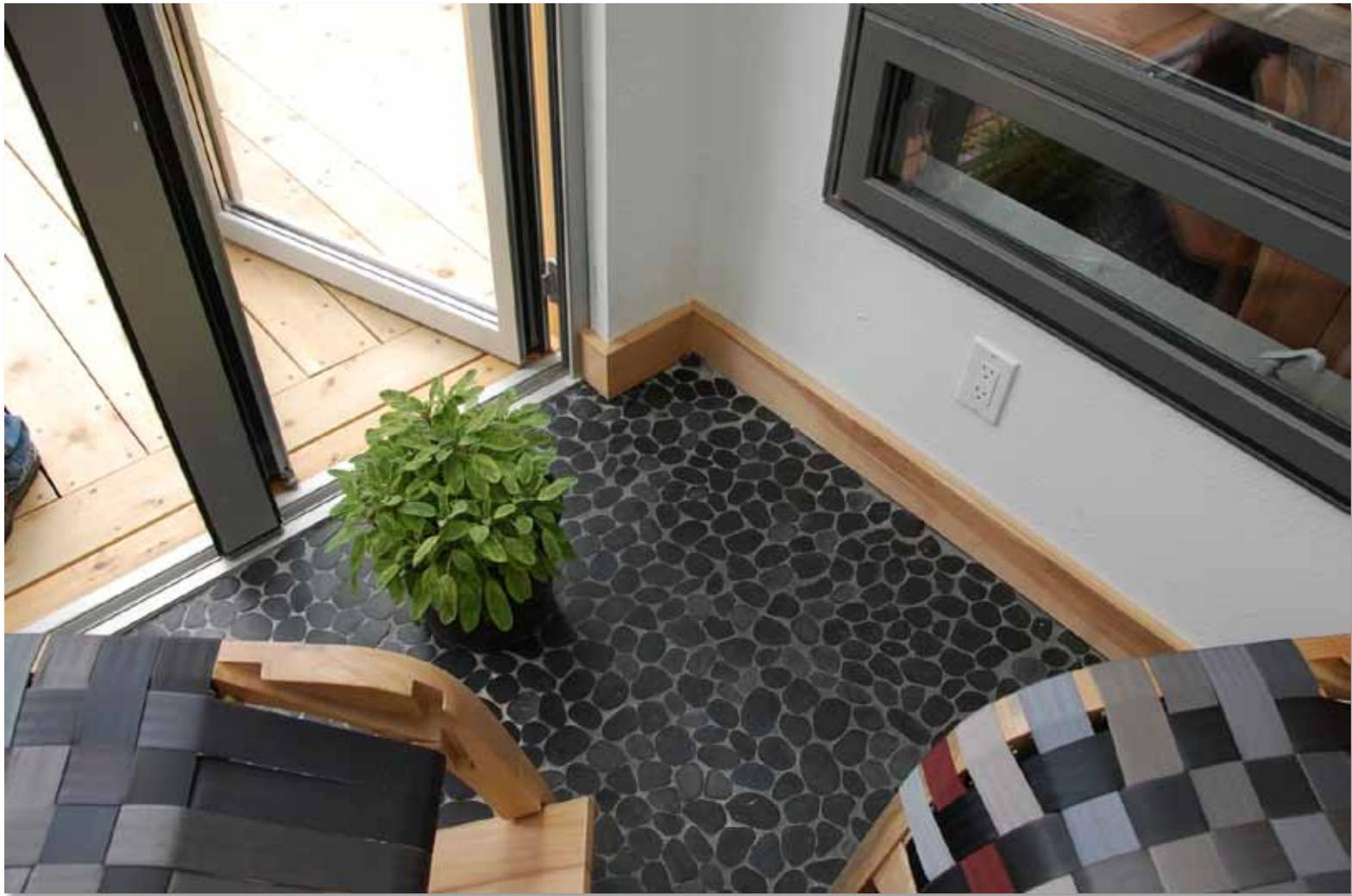
The floor of the sun space has thermal mass. Windows in the adjacent walls can be opened to allow the heat to enter.
