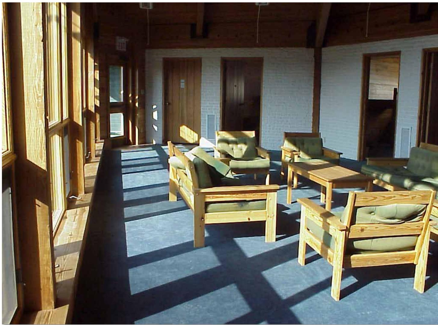
The white brick wall in the YMCA Burrows building is used to hold the heat that comes into the building through the windows. This is done in this wall, rather than in the floor (more usual), as the kids will be walking around in stocking feet.
