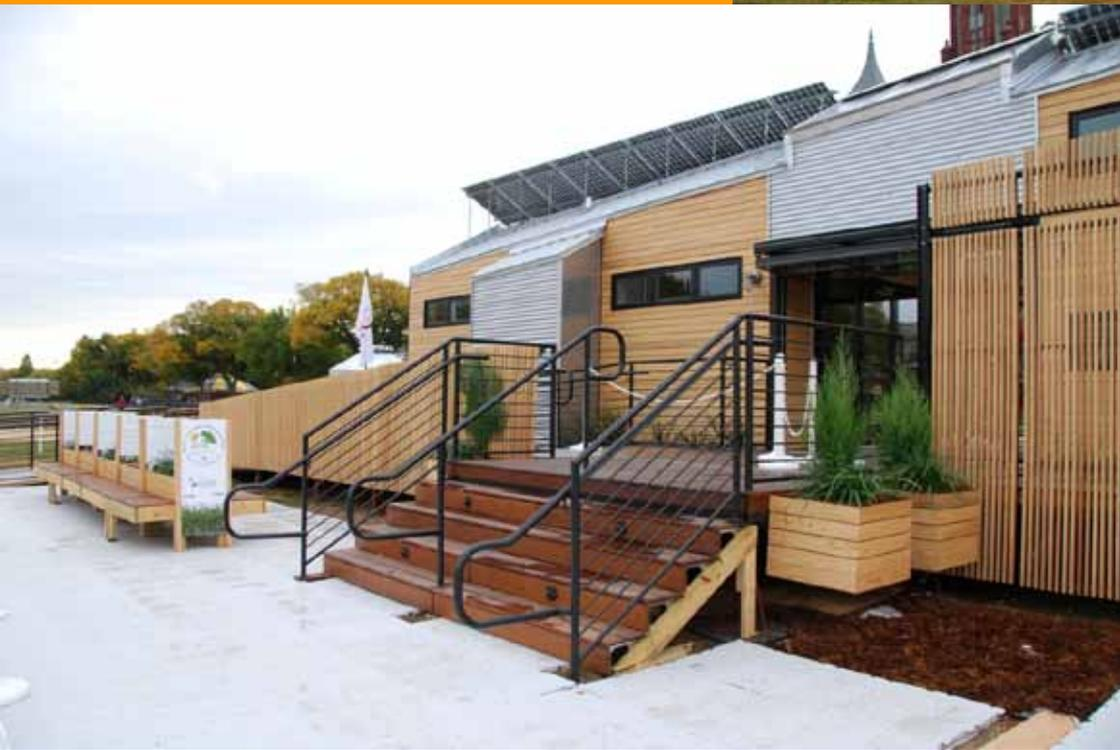
North face has small openings to minimize heat loss.
