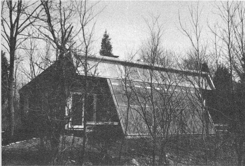
Figure 10.6: Solargreen exterior showing south-facing sunspace.
