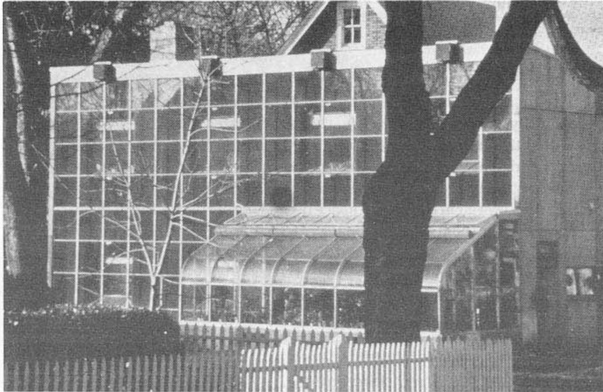
Figure 9.5: Kelbaugh house showing south facade with Trombe wall. (Photo courtesy of D. Kelbaugh.)
