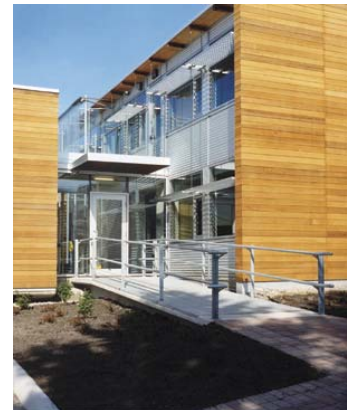
Main building entrance, Close-up view.
