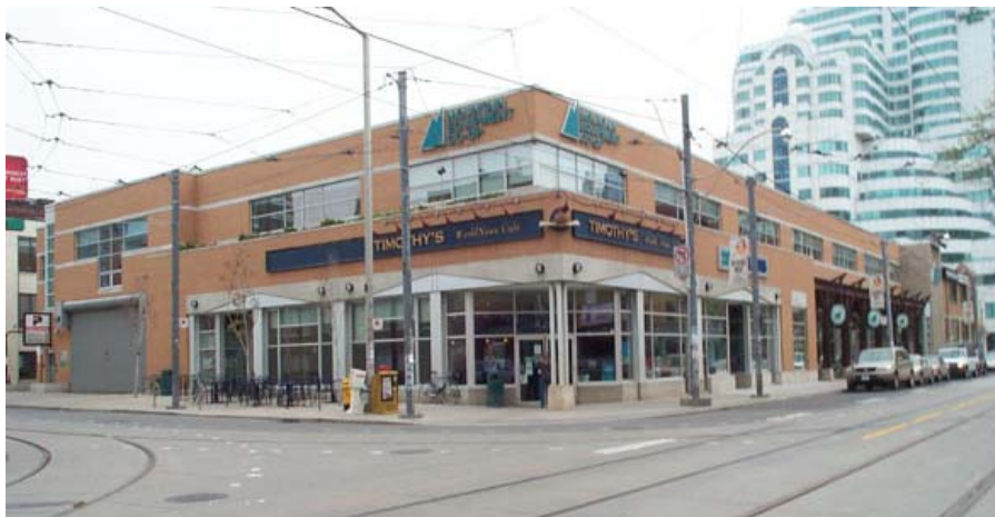
Charlotte Street Façade, with entrance to the underground parking garage at left, King Street Façade at right.
