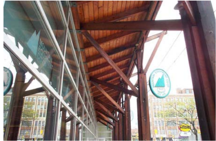
Covered bike area at entrance to building on King Street.
