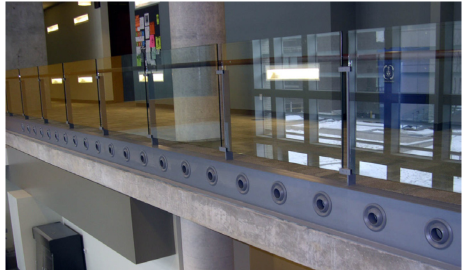
Figures 16 (Above Left): Air is drawn up the atrium using the stack effect. Figure 17 (Above Right): Vents at the top of the atrium. Figure 18 (Below): Diffusers are integrated into the floors slabs along the atrium walkways to aid in air circulation.
