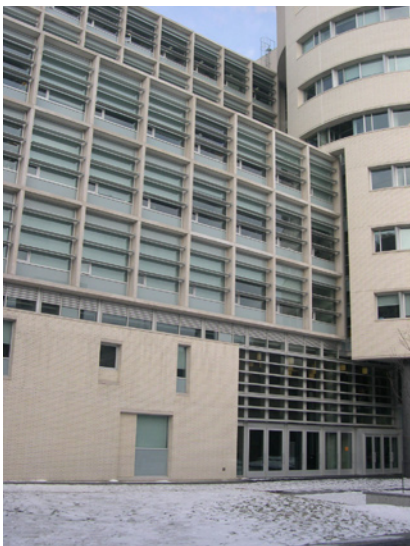
Figures 12 - 15 (Clockwise from Upper Left): Different facade treatments correspond to their exposure. Photos are west, north, south, and detail of the south louver system.
