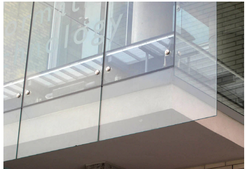
Figure 21 (Below): Detail of the Solarban Glazing at the main entrance of the building.
