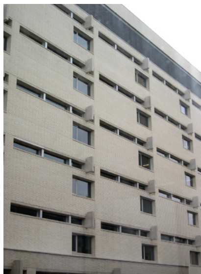
Figures 12 - 15 (Clockwise from Upper Left): Different facade treatments correspond to their exposure. Photos are west, north, south, and detail of the south louver system.
