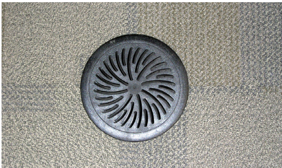
Figure 22 (Above): The water retention pond, seen here in winter, integrates storm-water management with aesthetics. Figure 23 (Below): The floor diffuser is one of the only visible signs of the ventilation system below the walking surface.
