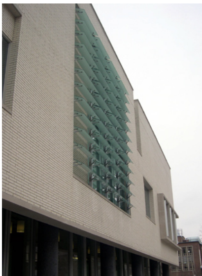
Figures 12 - 15 (Clockwise from Upper Left): Different facade treatments correspond to their exposure. Photos are west, north, south, and detail of the south louver system.
