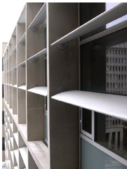
Figures 12 - 15 (Clockwise from Upper Left): Different facade treatments correspond to their exposure. Photos are west, north, south, and detail of the south louver system.
