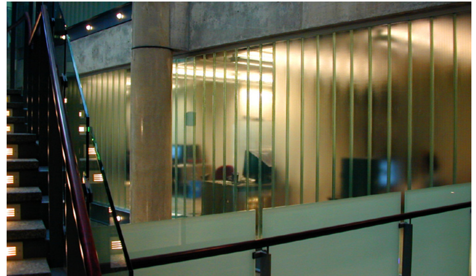
Figure 10 (Above): Interior partitions are low to allow light diffusion into spaces and moveable for increased flexibility. Figure 11 (Below): A glazed interior partition.
