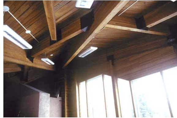
The glue-lam beams for ceiling.
