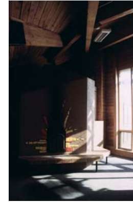
The masonry heater in the main room.
