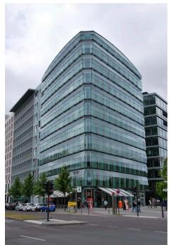
Fig 6: Double façade office building in Berlin, Germany. The exterior glass skin is not sealed and allows for migration of ventilating air to the interior while buffering noise. The interior façade is not fully glazed and includes opaque thermal elements with frequent operable windows.
