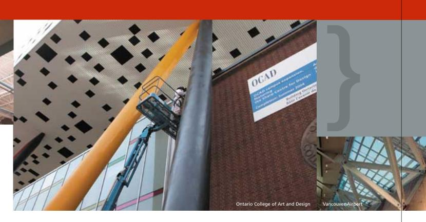
Intumescent coatings, although allowing exposed steel use in an increased number of occupancies, are not deemed by architects to be the best solution as they can result in a lumpy finish that can obscure some connection details. Fire protection methods for the exposed steel structure need to be determined early on as they should influence the type and design of connection detailing.
