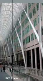
he modern application of steel in architecture has given way to a bold new set of manifestations. The exposed use of steel in design and construction has become a popular trend and method of architectural expression. Both standard steel shapes and steel tubes or HSS sections are being employed to create the architectural character of a building. This style is defined as *"Architecturally Exposed Structural Steel"* (AESS).
