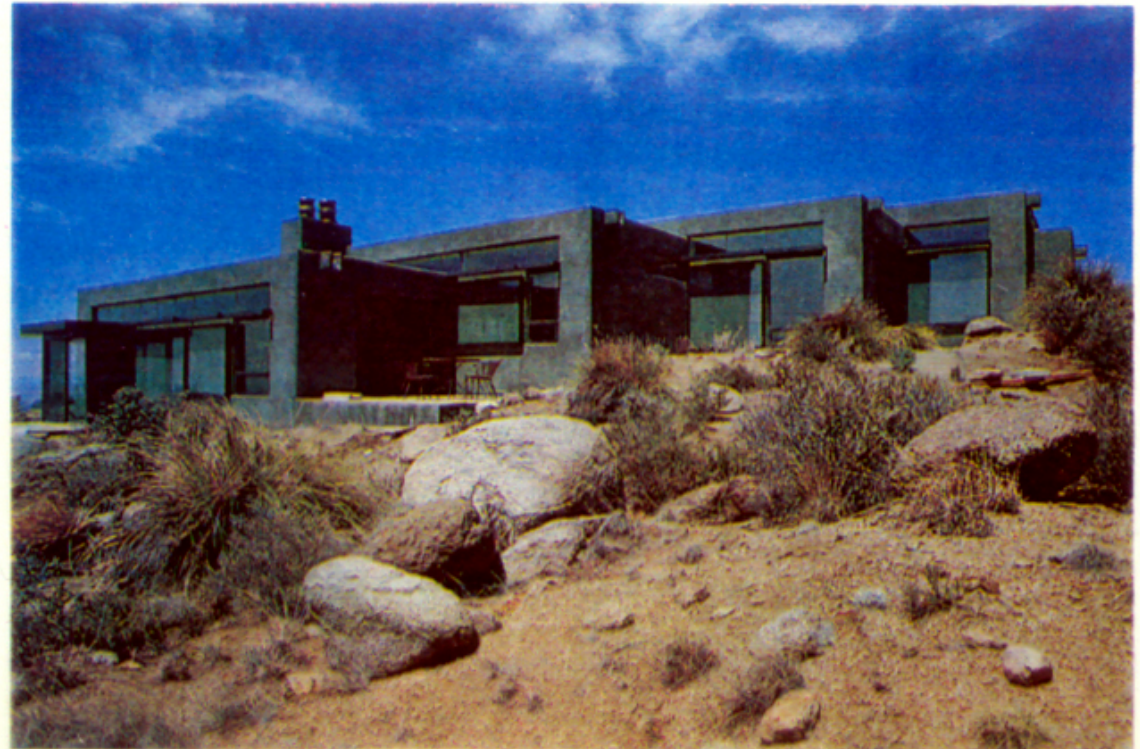
A view of the residence from the southwest (below). The non-vented trombe walls are visible on the south façade. The low winter sun strikes the trombe walls full strength (opposite).
