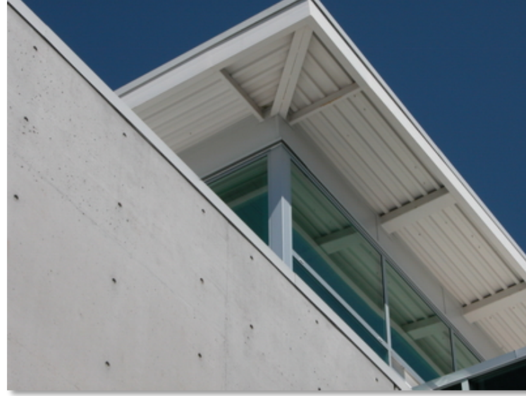
A simple roof overhang acts as a shading device.
