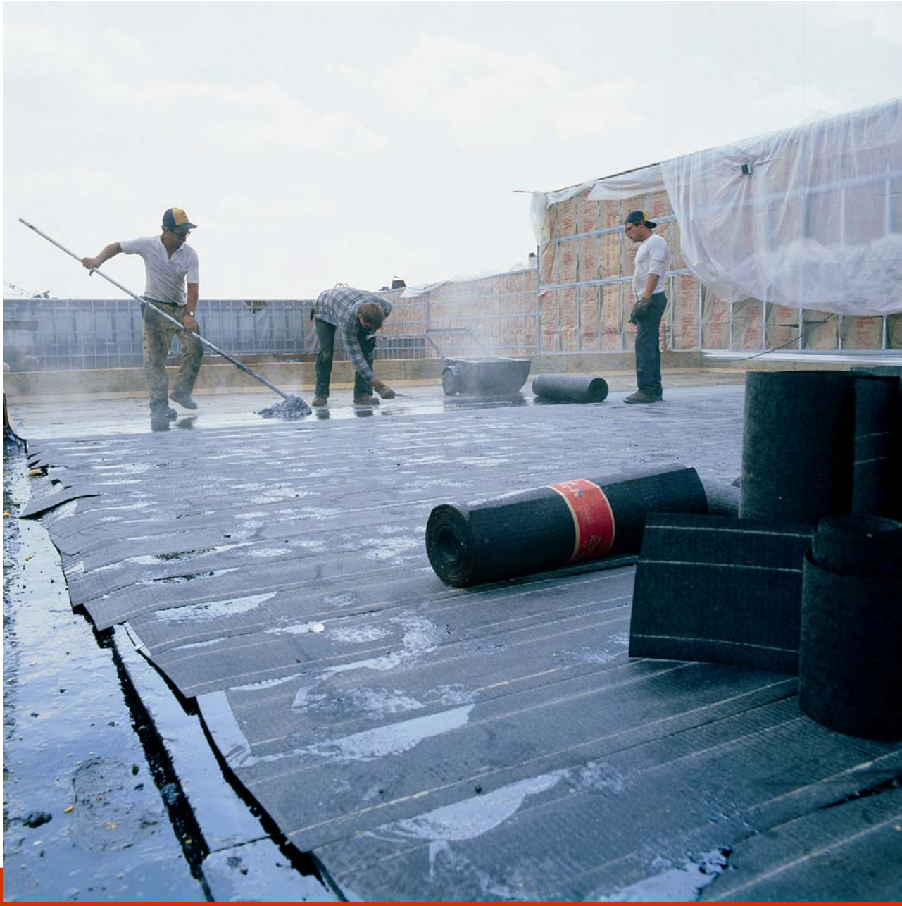
Built up Roof (BUR)
