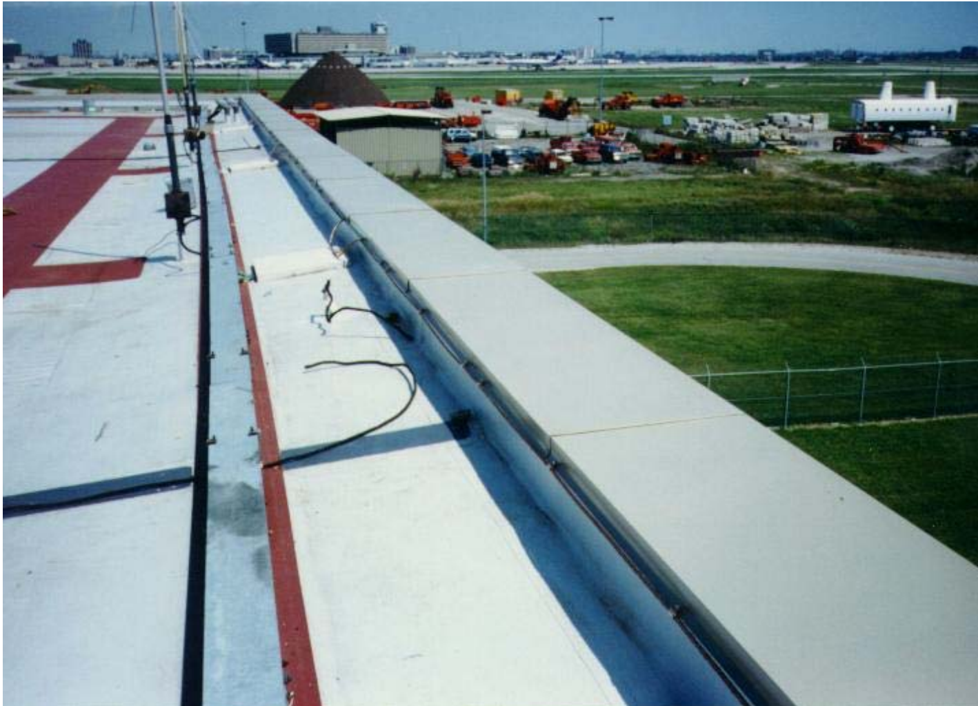
PVC Roof at Pearson International Airport
